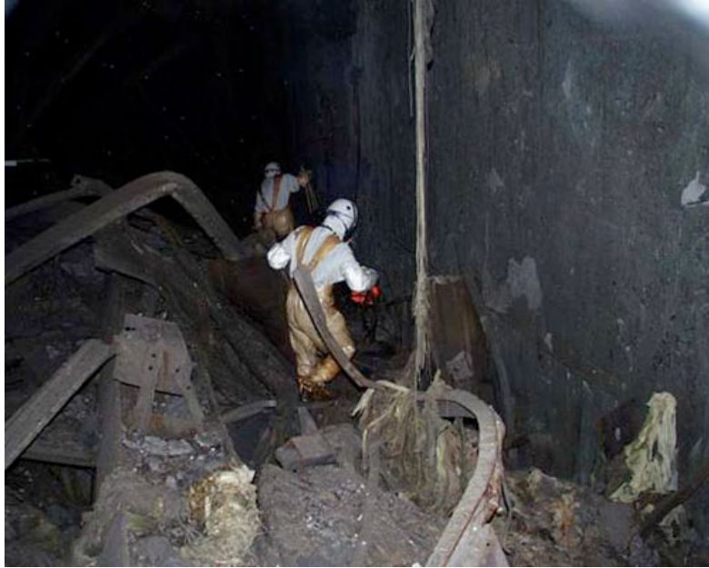
Figure 1. ChNPP personnel perform visual examinations in damaged areas of Unit 4 reactor to estimate FCM locations. Photo Credit: Chernobyl Center
